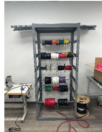
Electrical Wire Racking
